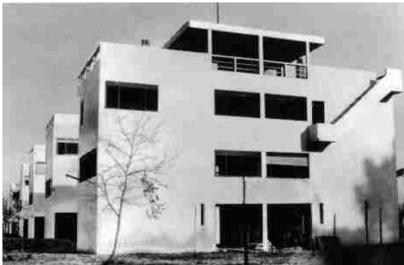
Figure 11: Housing at Pessac as originally built, 1924
