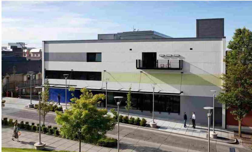
Figure 36: RFM renovated exterior
