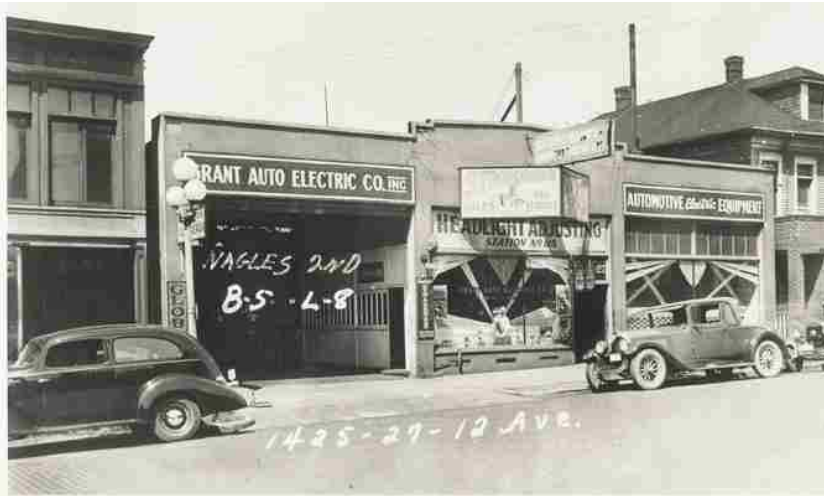
Figure 20: The Piston and Ring Building, before renovation
